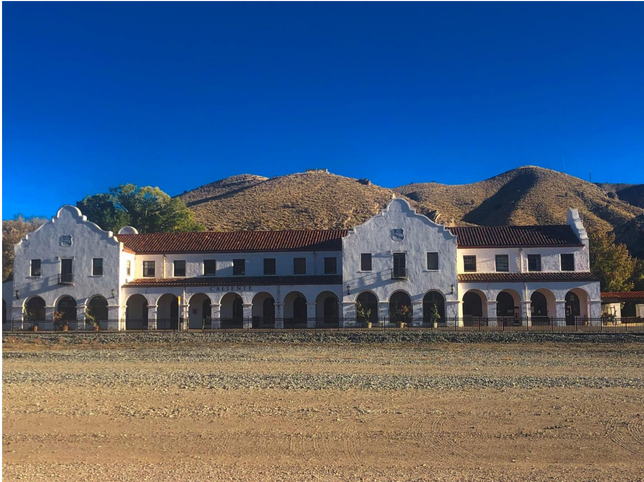
Caliente City Hall Station
