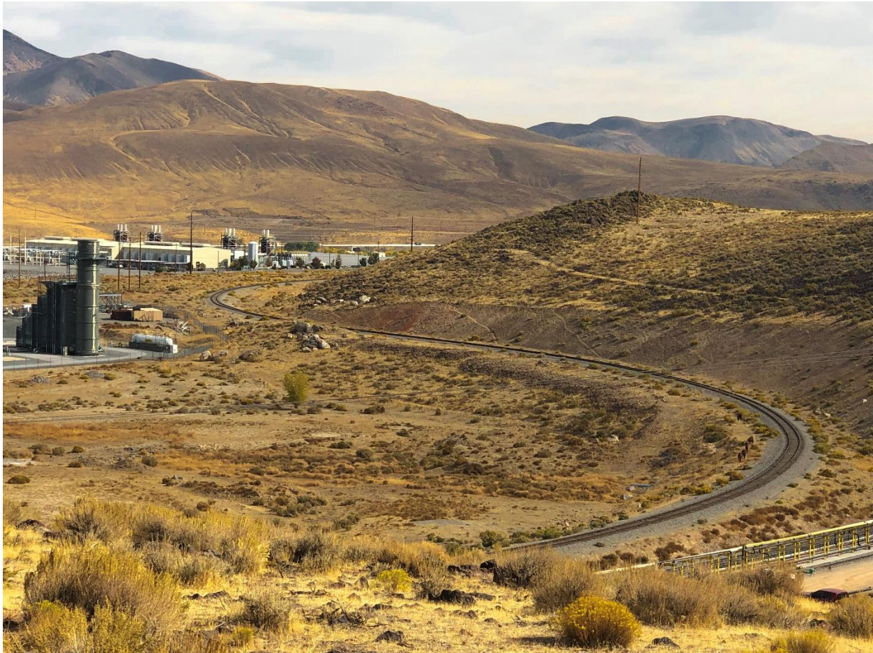
Branch line in the Tahoe-Reno Industrial Center
