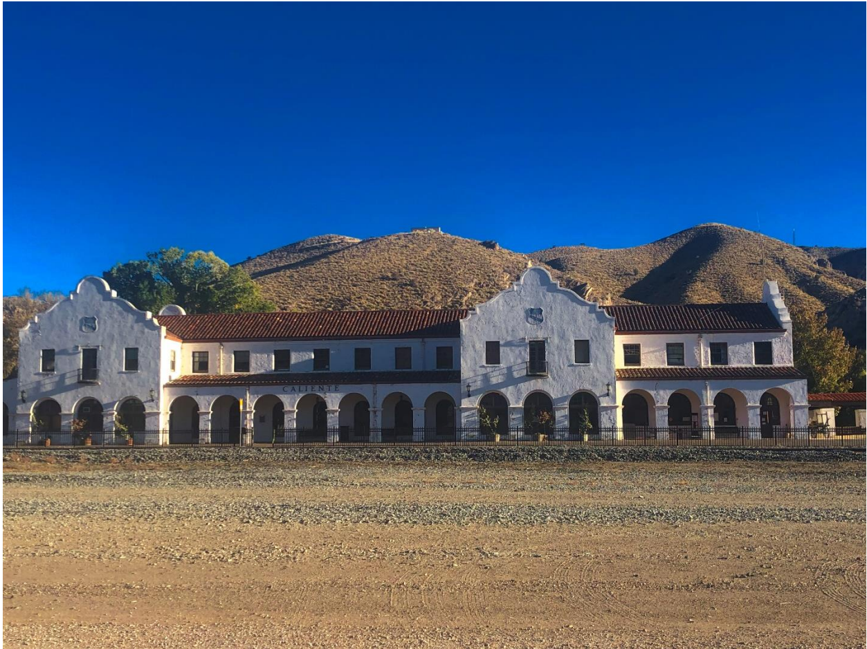
Caliente City Hall Station
