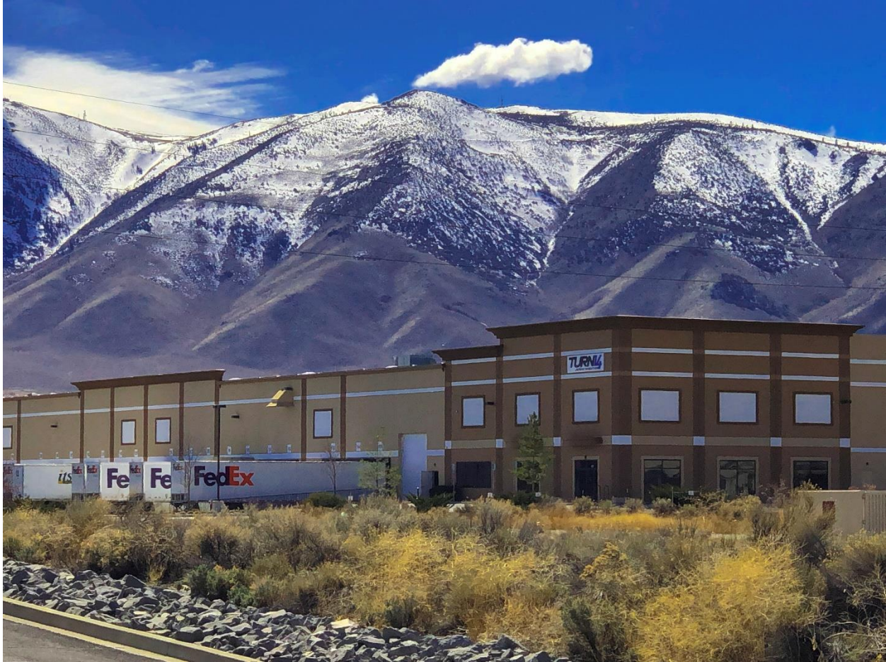
Stead Warehouse near rail line that does not use rail
